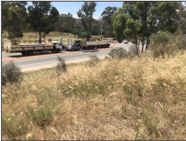
C-1. Looking southwards to Traffic lights. Need sign steep slope and tight corner.
